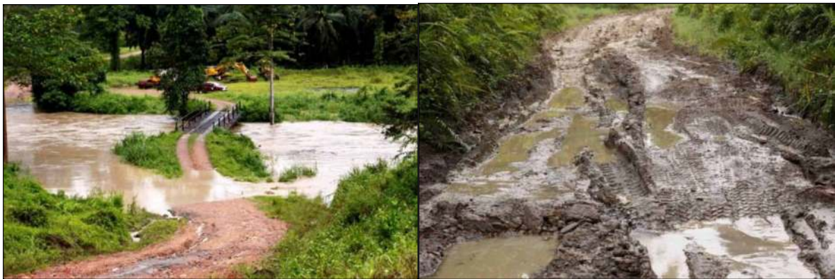
The usual dry period which occurs at some time between February-April in Tabin failed to occur in 2011, with rain on most days through the period. (Figure 4, left) Lipad river at Tabin HQ flooded on 9 April, (Figure 5, right) road to the interim rhino paddocks, April, where the condition became almost impassable and was repaired temporarily, manually and with assistance of an excavator.
