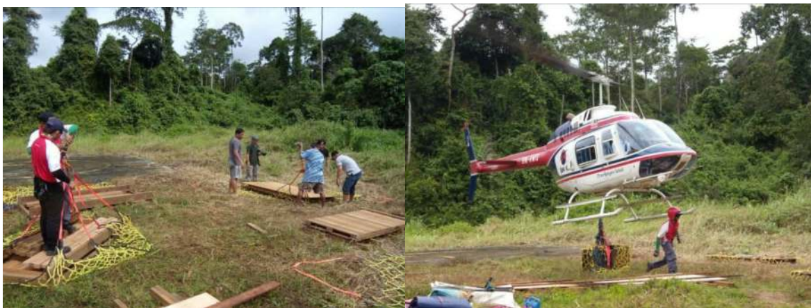
(left) preparation of materials to be brought to the Malambabula site for construction of a third and fourth trap for Puntung, (right) air lift of materials to the third and fourth trap site (20 December)
