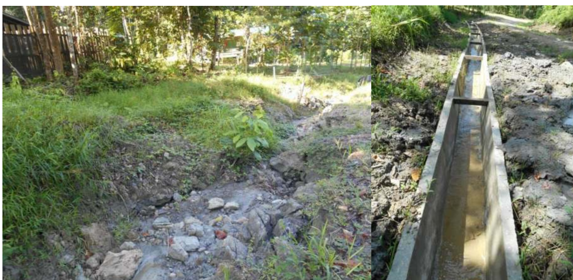
Road next to the interim rhino facilities at Tabin, (left) a drain dug in 2012 eroded to this by July 2013, (right) the concrete roadside drain completed in early October
