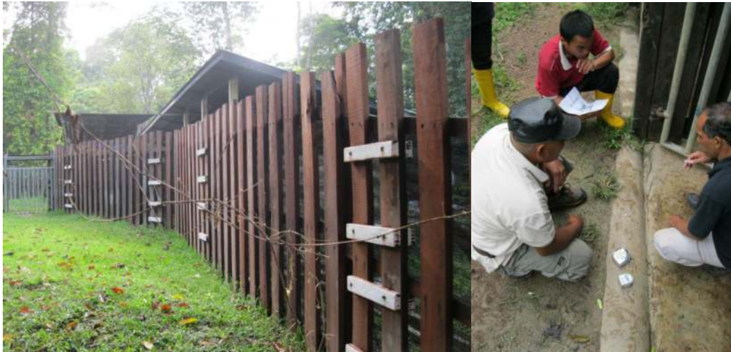
(left) rhino breeding yard, with added emergency keeper escape ladders in case of aggressive behaviour by Tam, (right) measuring for replacement of a swing door with a sliding door
